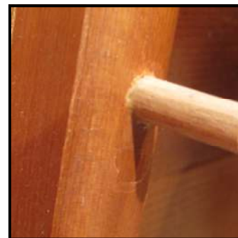
Dowel inserted in place.
